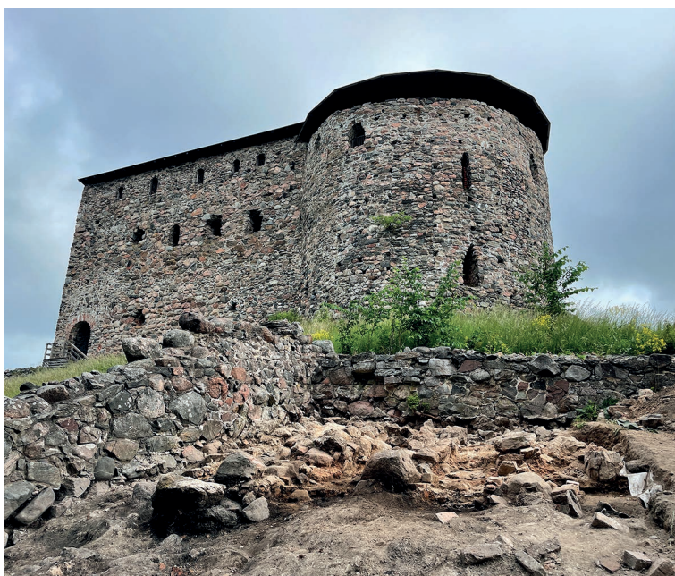
FIGURE 8. General view of the kiln and the Raseborg Castle. Photo: Majja Holappa.
