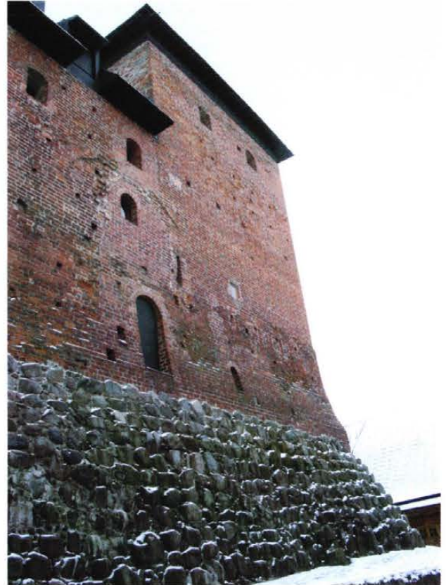
Figure 10. Going from Häme Castle's main structure into the fatabur tower was arranged practically. Very few remnants of the fatabur tower have been preserved, but on the wall, at a height of about 5 meters, is a door opening that still reminds us of the fatabur: from the main castle's second level, a wooden bridge led, at that time, directly into the fatabur tower. Photograph Terhi Mikkola. (NBA, Häme Castle)
