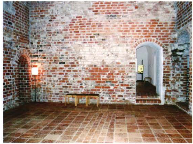
Figure 20. The eastern gable of the Northeast wing. On the left is a door to the Dansker tower. On the right, a door to the gallery on the level of the first floor. From that door passage, as from the door in the middle, rose a stairway to the upper parts of the castle. Photograph Terhi Mikkola. (NBA, Häme Castle)
