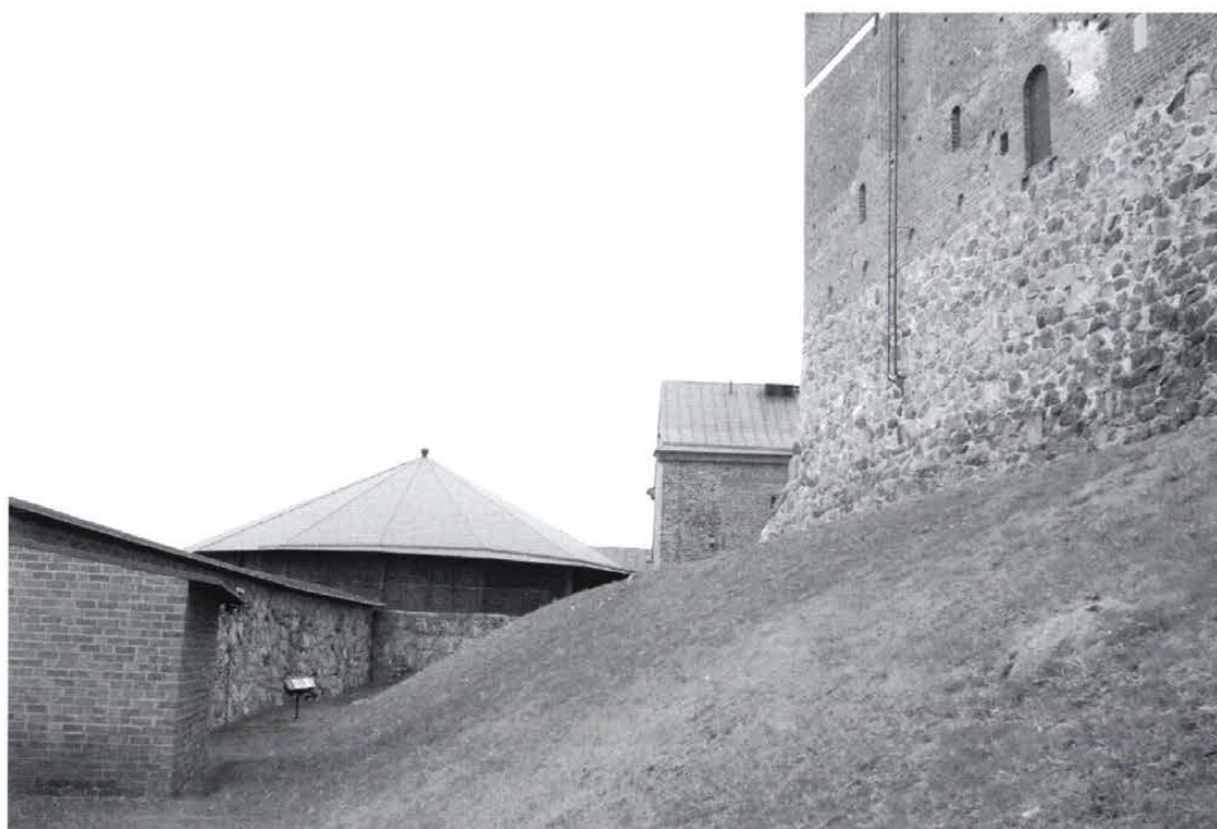
Figure 27. View toward the current northeastern outer ward. In the background is the rondel and on the left the curtain wall beside the lake Vanajavesi. In the wall of the castle, just above the greystone masonry, is the door that led to the bridge between the Northeast wing and the Dansker tower in the curtain wall. Photograph Martti Lampila. (NBA, Häme Castle)
