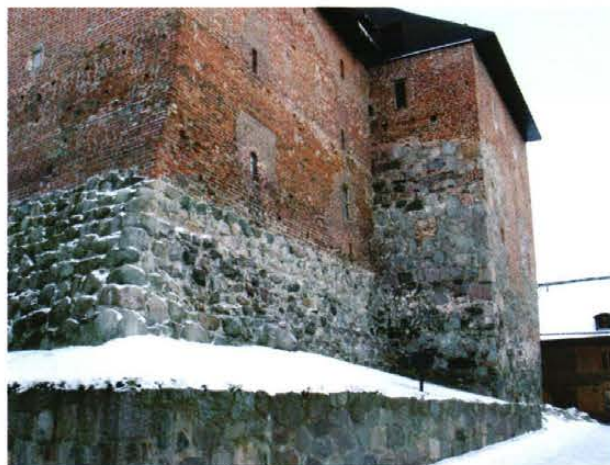
Figure 15. The Cock tower protruding from the Southwest wing of the castle. Photograph Terhi Mikkola. (NBA, Häme Castle)
