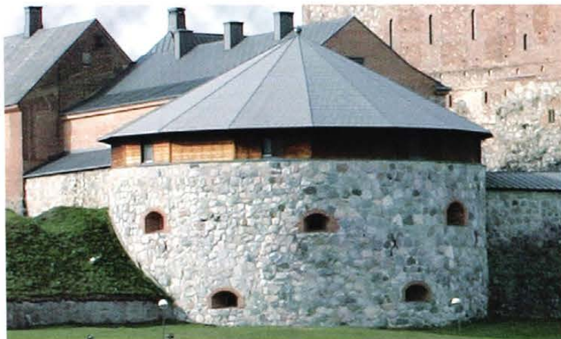
Figure 11. The eastern gun tower, or rondel, built during the year 1559, is the only structure from the Vasa period preserved at Häme Castle. The tower was built low, and apparently there were originally only two levels. It was roofed. The current roof was completed in 1983 in connection with the castle's restoration. On the right side of the rondel is preserved part of the medieval curtain wall. Photograph Martti Lampila. (NBA, Häme Castle)
