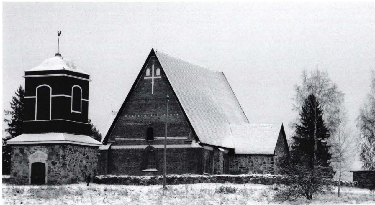
Figure 39. Hattula Church from the southwest. Photograph Terhi Mikkola.
